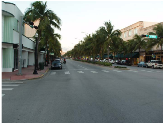
Figure 3. Street view of Washington Avenue.
